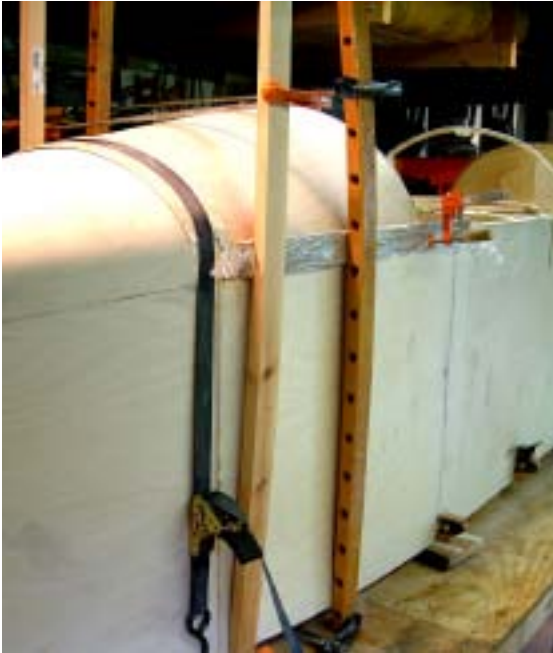
Straps were invaluable for holding the decking in place.
